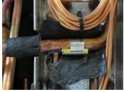
6. Remove the sensor from the suction line and cut the wire as close as possible to the drain pan.
