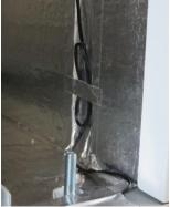
12. Use metal tape to secure the wire to the base, drain pan and inlet panel.
