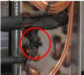
5. Remove the cork tape from the sensor on the suction line.
